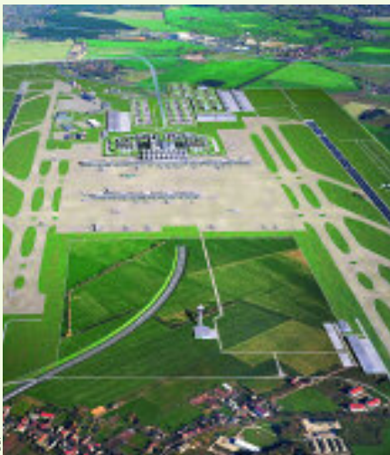
A total of 7.5 million euros will be invested in business aviation infrastructure at Berlin's new airport hub
